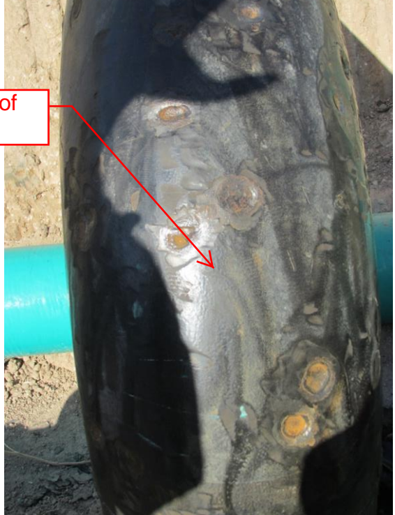
12-inch 90 degree elbow to be replaced
